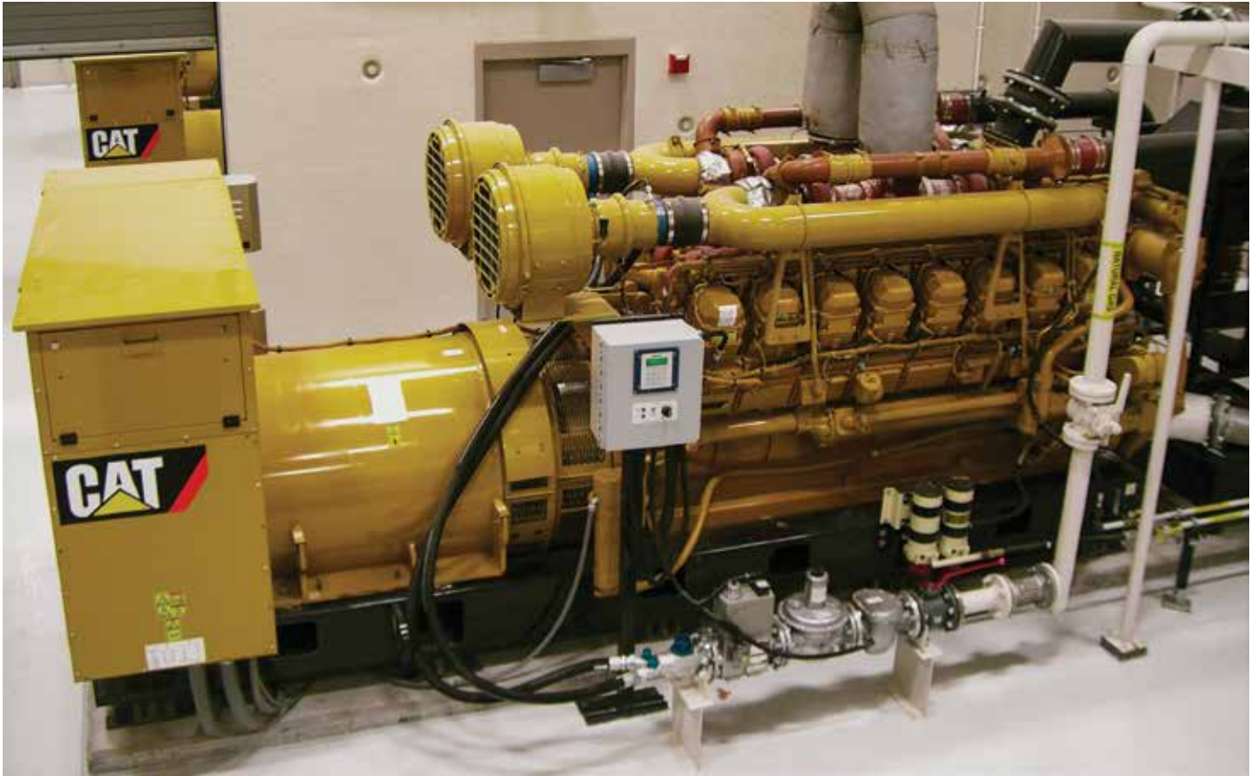
Water Treatment Facility
